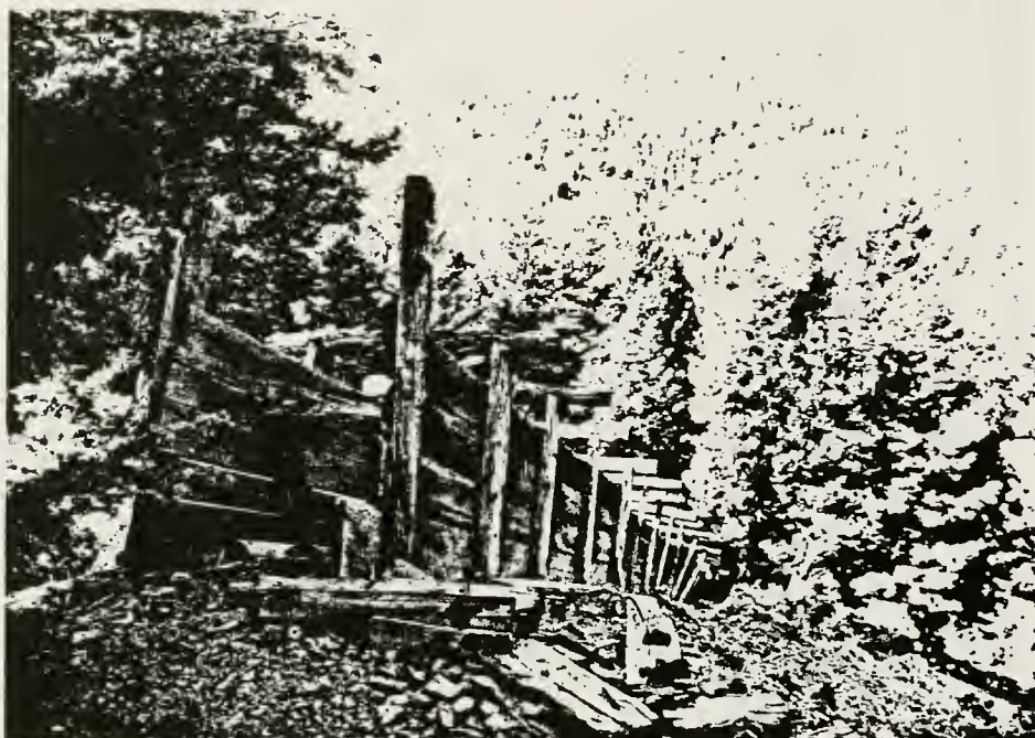
Figure 243. Feature #134, top of gravity ore chute standing on waste dump, west view.
